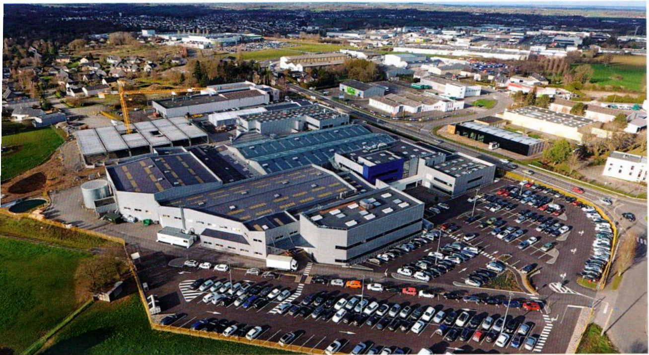
GYS' main factory and R&D centre in Laval, France
